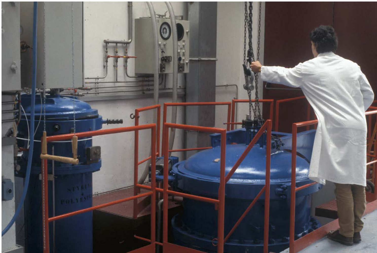
Impregnation tanks 200 litres (left) and 3000 liters
