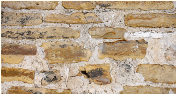
Detail of the wall made of sedimentary rocks – flysch (V. Marinković)
