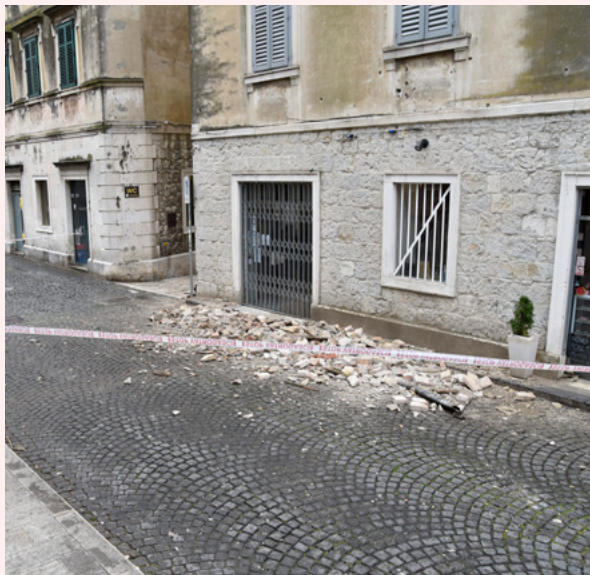
The roof cornice collapsed due to the 2021 heavy rain (J. Šupić / Cropix)
