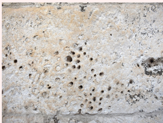
Deterioration of stone (V. Marinković)
