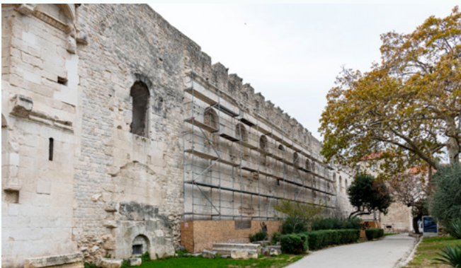
Scaffolding must satisfy the rules, regulations and standards of protection (P. Gamulin)
