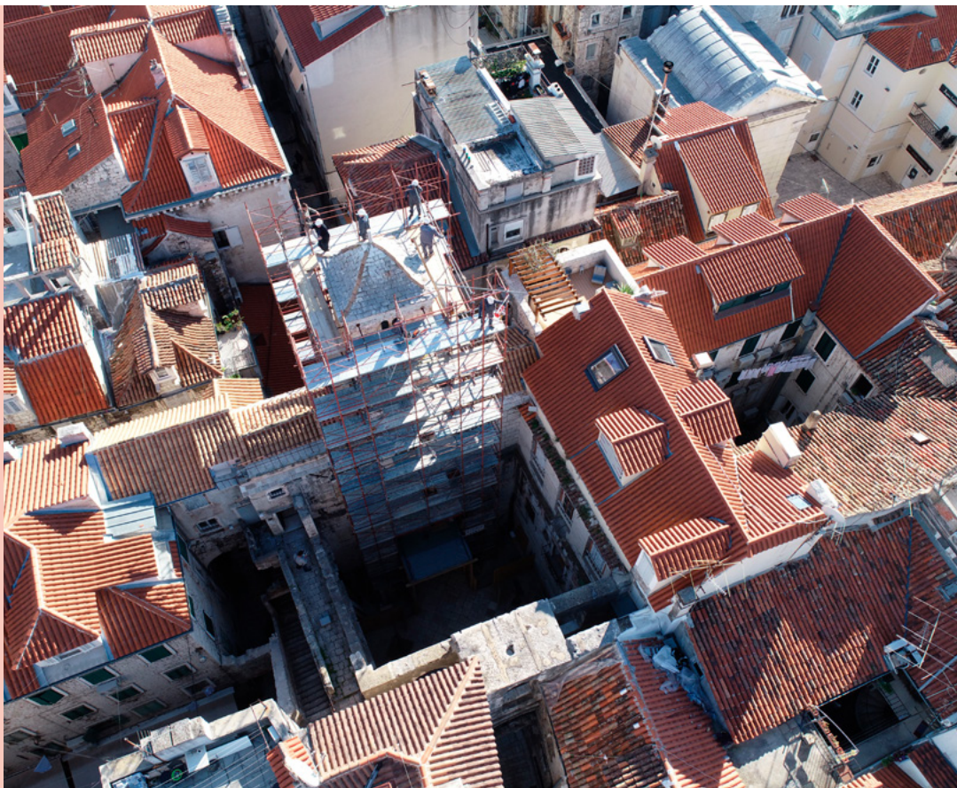
Restoration works on the bell tower of the church of Gospe od Zvonika (archives of the Croatian Conservation Institute and Geoprojekt d.d.)
