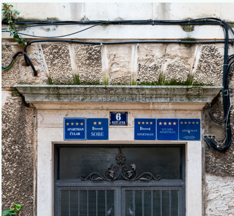
Pursuant to the Order on the Communal Order , it is prohibited to put signs on stone frames of the openings in the protected Zone A (V. Marinković)
