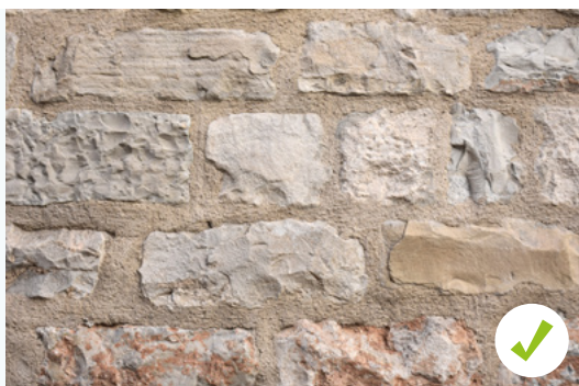
Correctly grouted lime mortar joint (V. Marinković)
