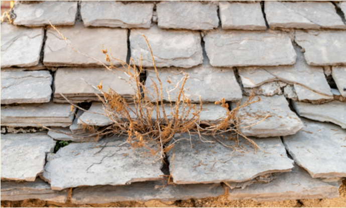
Detail of the stone roof (P. Gamulin)
