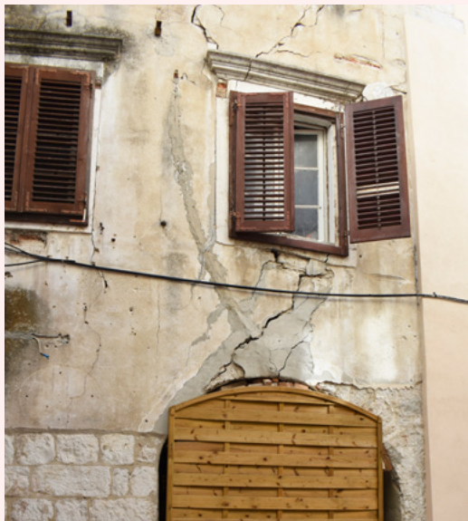
Structural damage on a house in Bulić Street, such constructions are extremely vulnerable to earthquake (V. Marinković)
