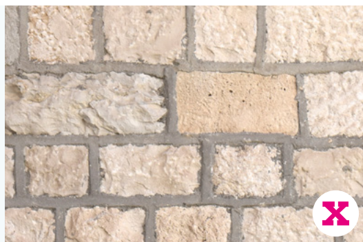
Incorrectly grouted joint: inadequate material and treatment (V. Marinković)
