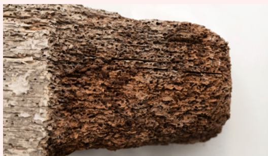
A damaged timber joist (P. Gamulin)
