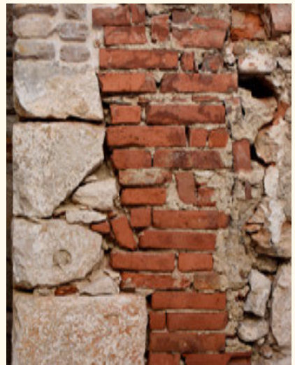
Detail of brick and stone masonry (V. Marinković)
