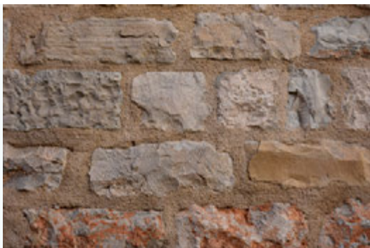
Correctly grouted lime mortar joint (V. Marinković)
