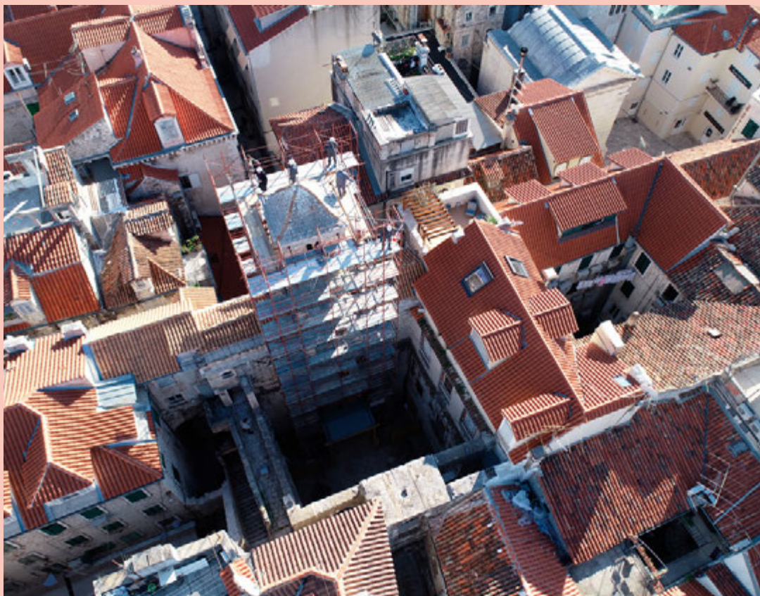
Restoration works on the bell tower of the church of Gospe od Zvonika (archives of the Croatian Institute for Restoration and Geoprojekt d.d.)
