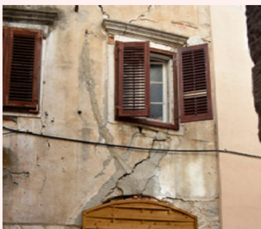
Structural damage on a house in Bulić Street. Such constructions are extremely vulnerable in an earthquake (V. Marinković)
