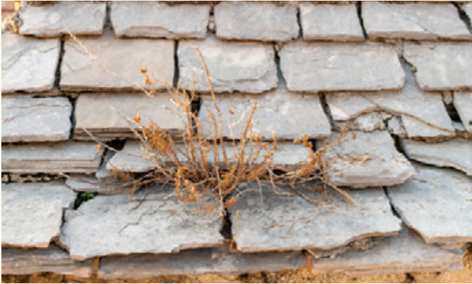
Detail of the stone roof (P. Gamulin)
