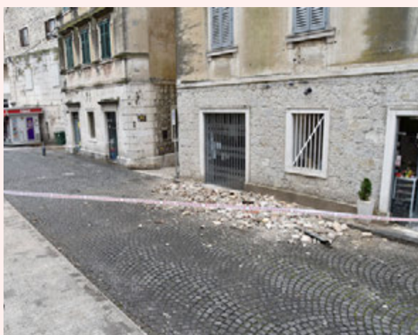
The roof cornice collapsed due to the 2021 heavy rain (JoškoŠupić/ Cropix)
