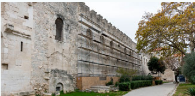
Scaffolding must satisfy the rules, regulations and standards of protection (P. Gamulin)
