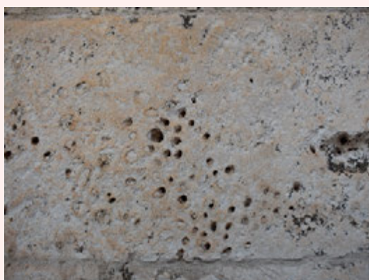
Deterioration of stone (V. Marinković)
