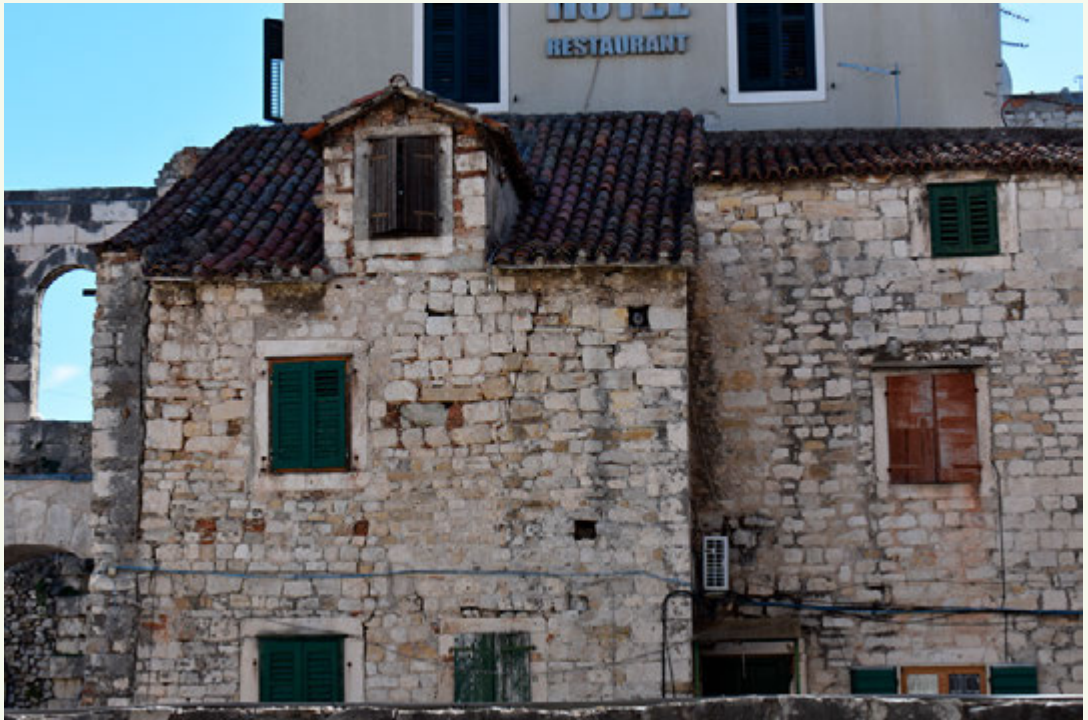
Detail of old house in Bulić Street (V. Marinković)
