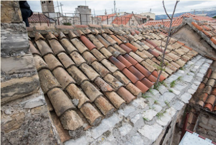
Detail of the roof containing remains of the old stone roofing and the new barrel tiles (N. Vasić)
