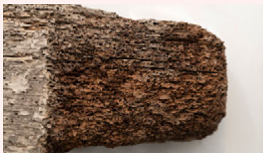
A damaged timber joist (P. Gamulin)
