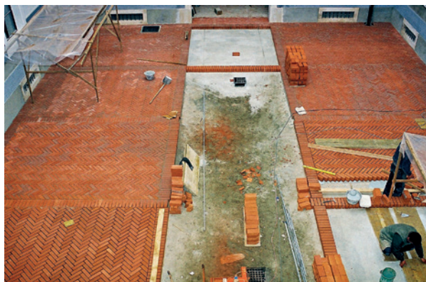
Postavljanje opeke u dvorištu / Laying the bricks in the courtyard
