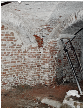
Saniranje zidova u podrumu Improvement of walls in the basement
