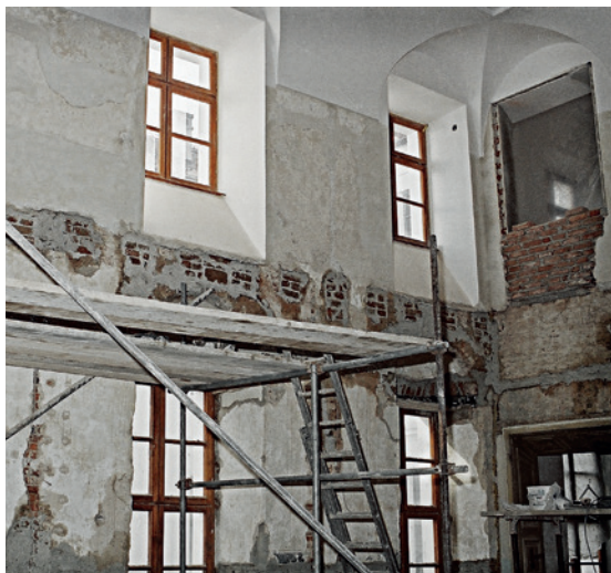
Građevinski radovi u svečanoj dvorani Construction work in the great hall
