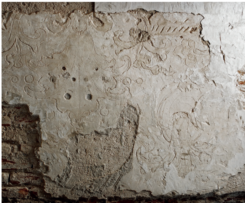
Fragment barokne žbuke s sačuvanim gravurama za štukature u svečanoj dvorani Fragment of the Baroque-period plaster with the preserved drawings for stucco-decorations in the great hall
