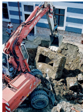
Iskop betonskih elemenata u dvorištu Concrete elements dug out in the courtyard
