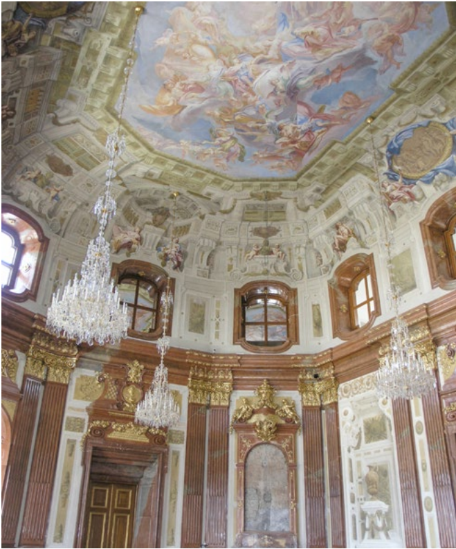
Marble Hall in the Upper Belvedere, Vienna, after restoration. The structure was heavily damaged in 1944. (BDA Archive, photo: Tinzl, 2005)
