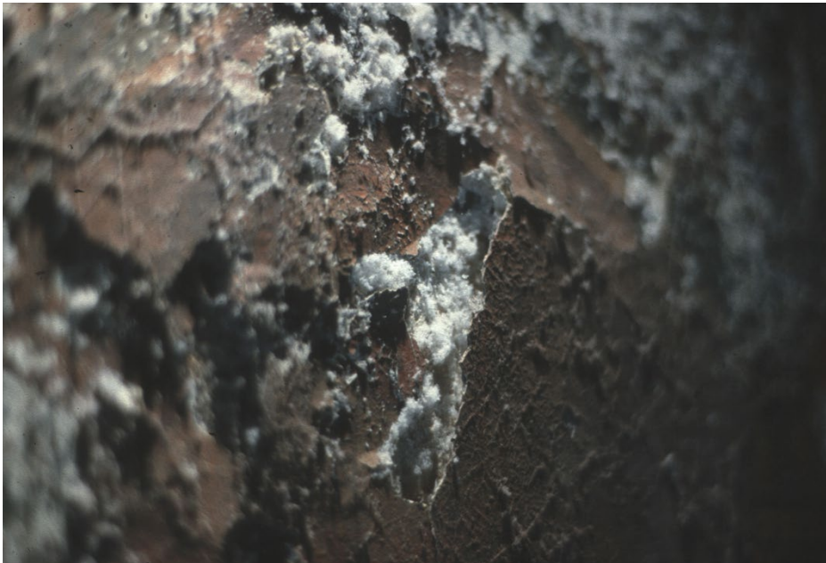
| Climate controlled salt crystallization on wall paintings in Neustadt/Mußbach, Rhineland-Palatinate, Germany Klimatski kontrolirana kristalizacija soli na zidnim slikama u Neustadtu/Mußbachu, Rhineland-Palatinate, Njemačka
