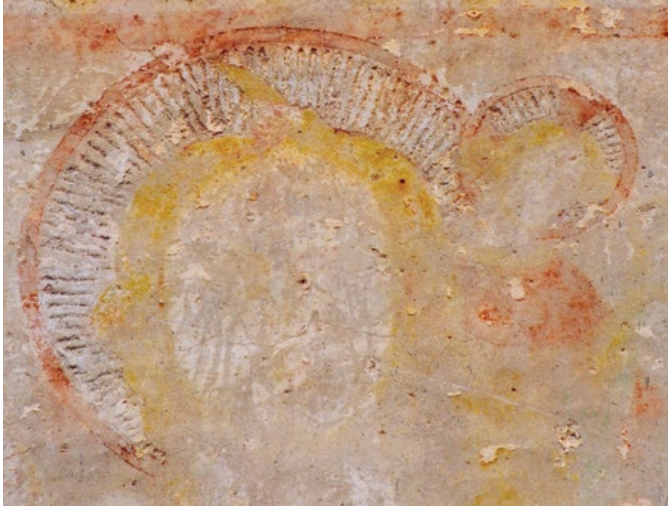
| Pitting decay and colour fading occurring on wall painting on the exterior of St. Thomas's church in Velike Poljane, Slovenia Jamičasto propadanje i blijedenje boje na zidnim slikama na fasadi crkve sv. Tome u Velikim Poljanama, Slovenija
