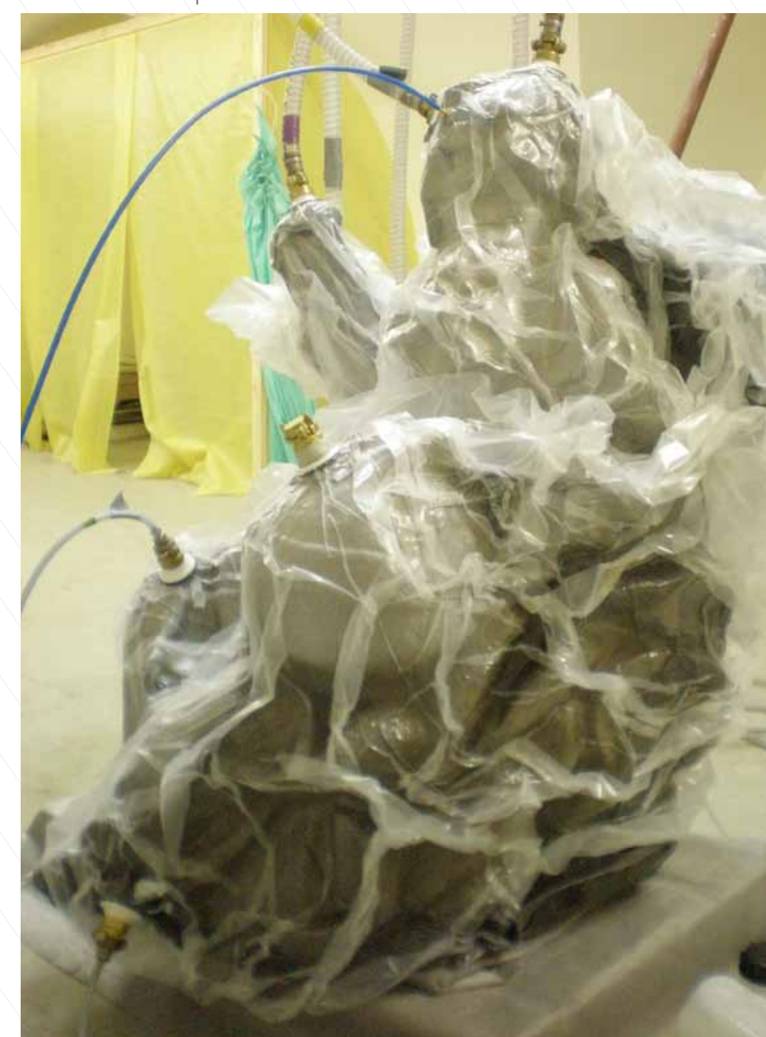
Vakuumsko učvršćivanje skulpture Boga Oca u radionici Vacuum reinforcement of the statue of God the Father in the workshop
