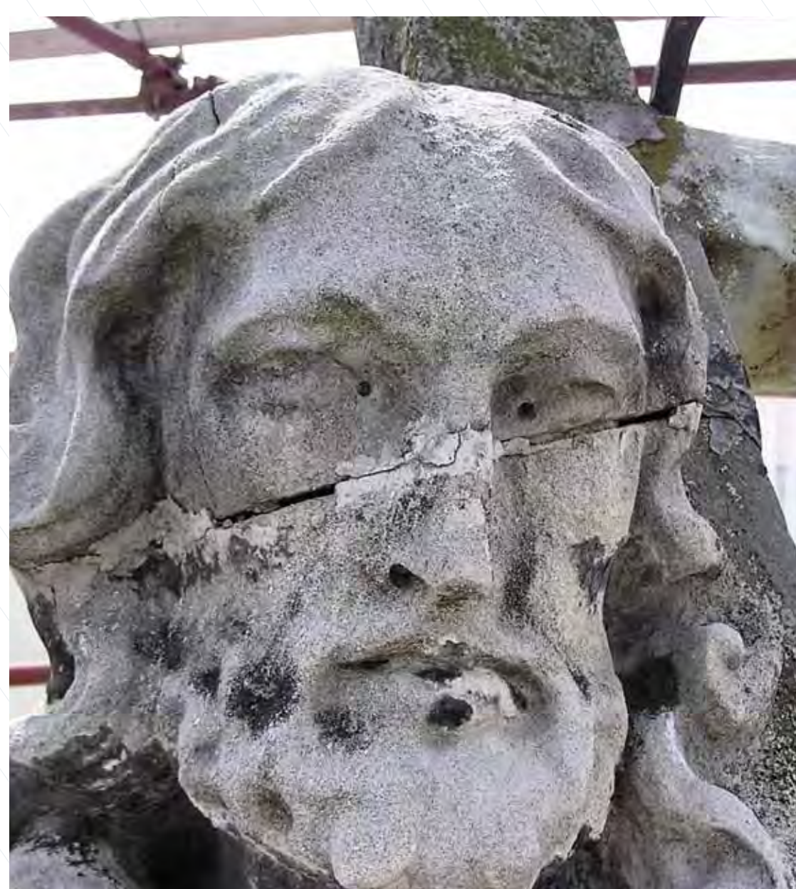
Oštećenja kamena na glavama skulptura: anđela, Boga Oca, Krista i sv. Josipa Damages of stone on the heads of an angel, God the Father, Christ and St. Joseph
