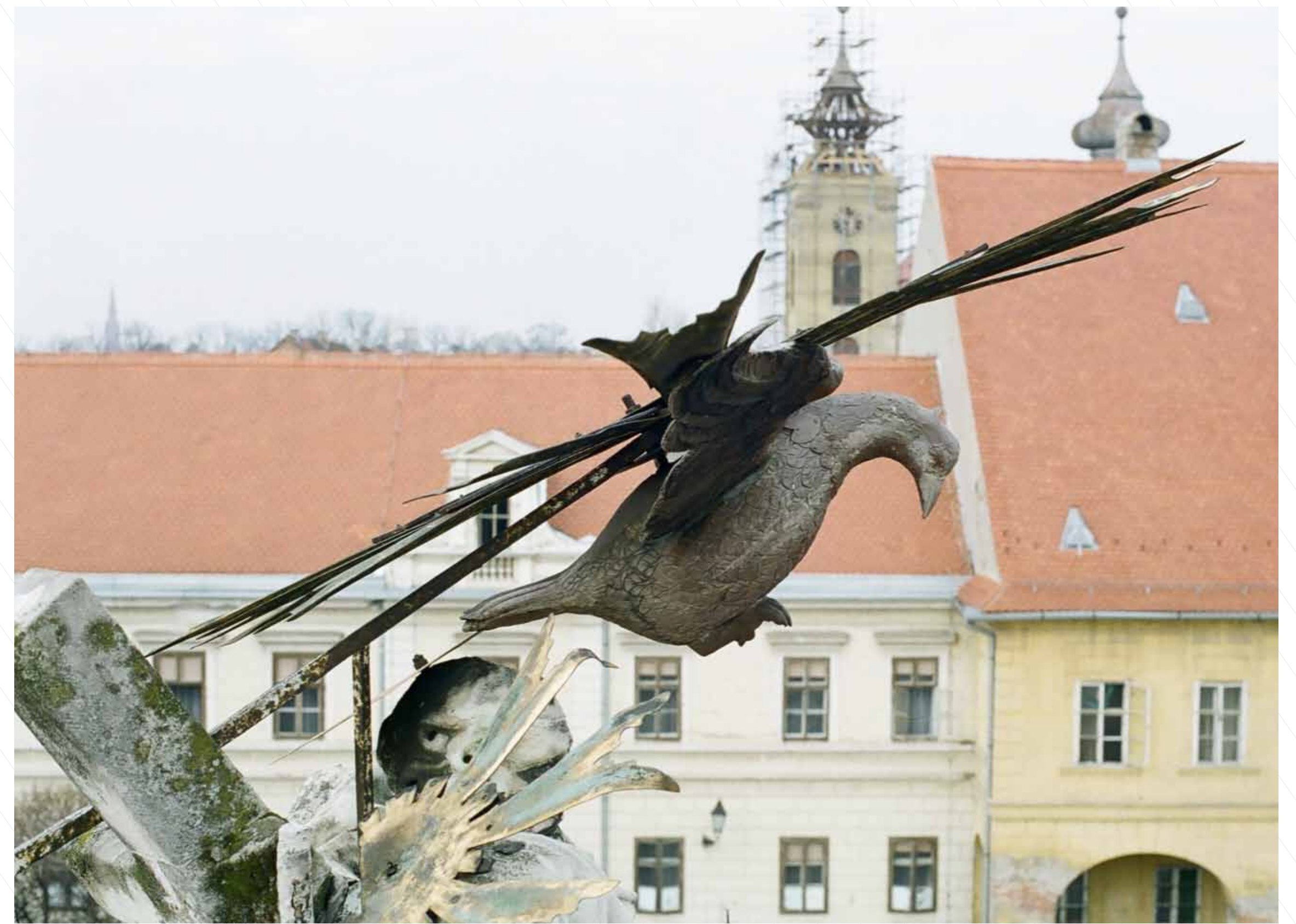
Poliesterska kopija golubice postavljena tijekom restauratorskih radova 70-ih godina Replica of the dove made of polyester during the restoration work in the 1970s
