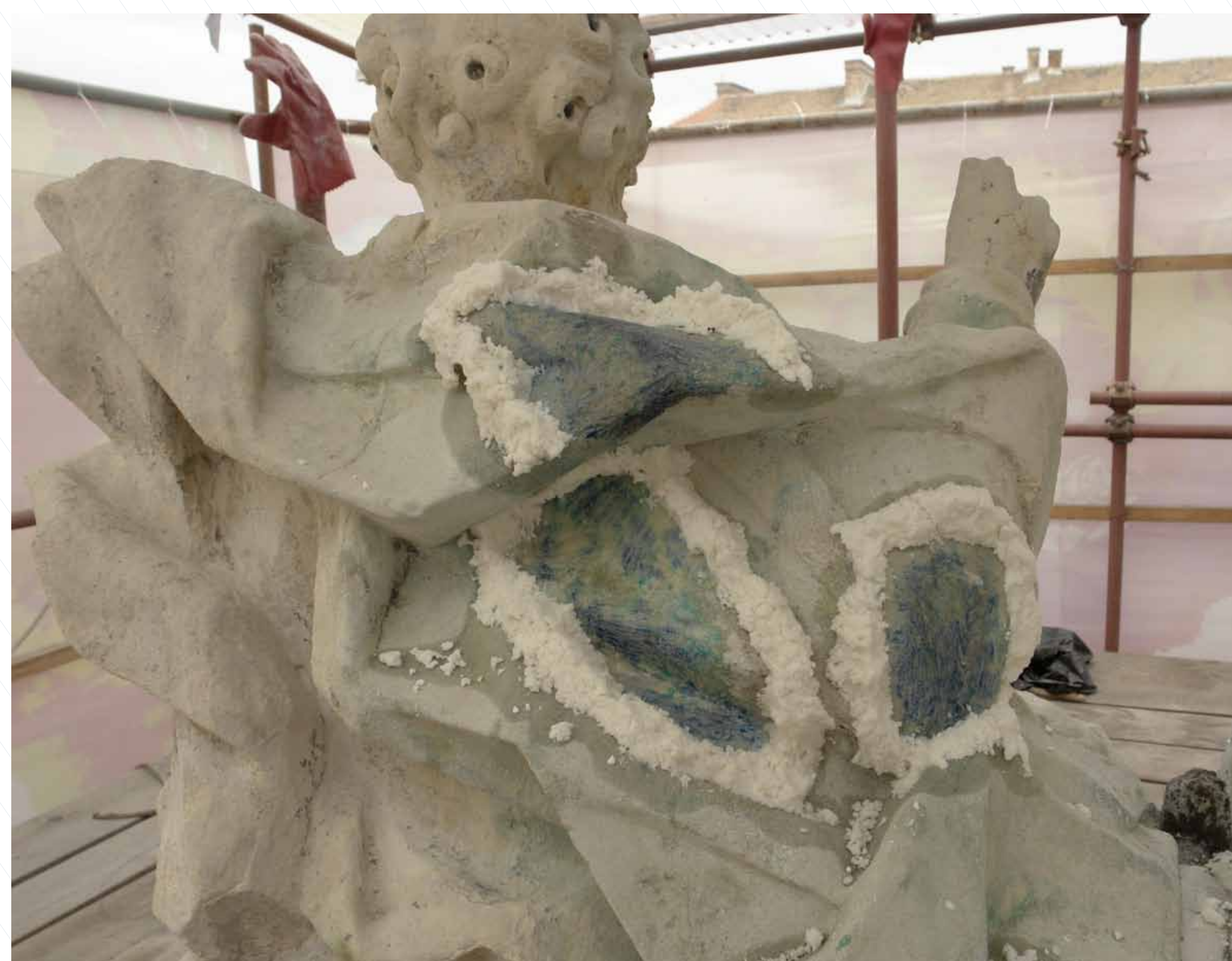
Uklanjanje malahitnih mrlja sa skulpture Boga Oca pulpom natopljenom amonijevim karbonatom Removal of malachite stains from the statue of God the Father by pulp saturated with ammonia carbonate
