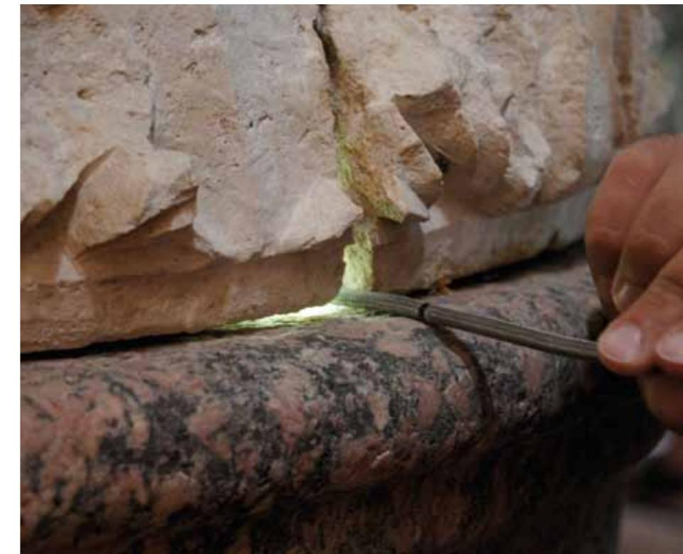
ENDOSKOPSKO ISPITIVANJE ŽELJEZNOG TRNA IZMEĐU GRANITNOG STUPA I KAPITELA NA PROTIRONU
