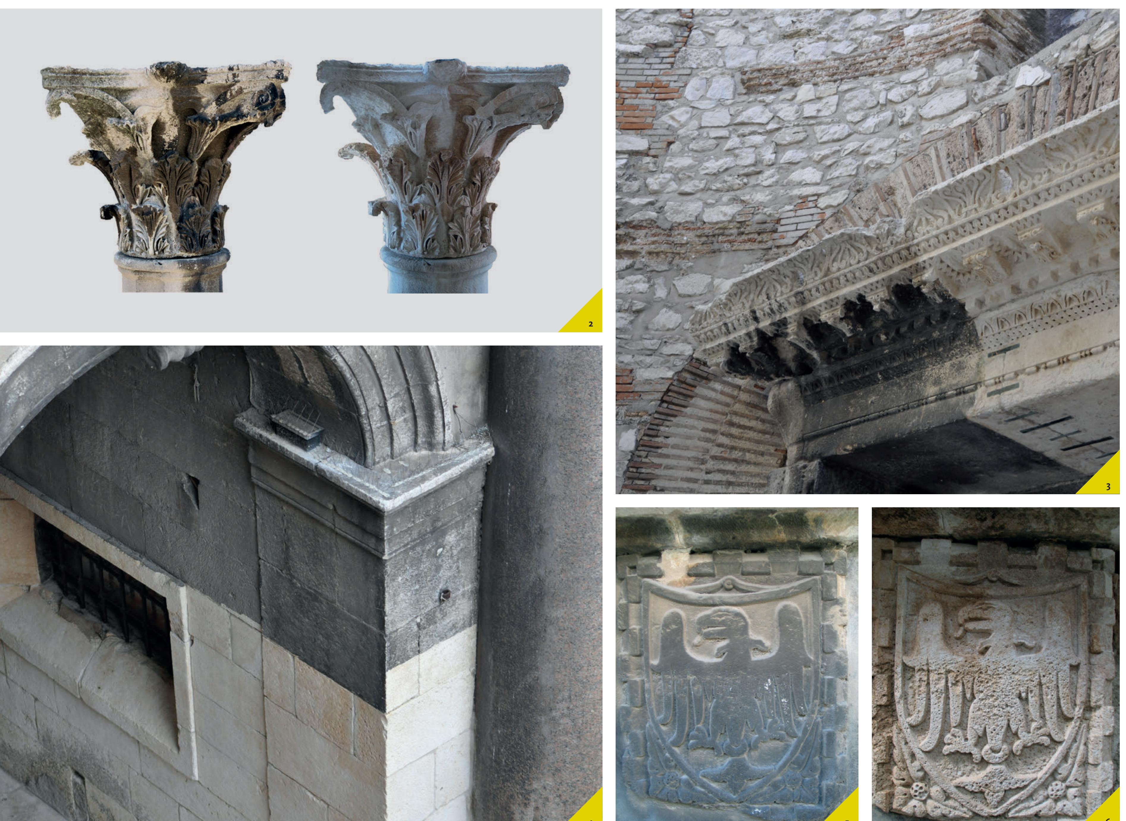
1. ČIŠĆENJE KAMENA LASERSKOM TEHNOLOGIJOM; 2, 3, 4, 8. USPOREDBE OČIŠĆENIH I NEOČIŠĆENIH ZONA; 5, 6. GRB OBITELJI GRISOGONO PRIJE I NAKON LASERSKOG ČIŠĆENJA; 7. LASERSKO ČIŠĆENJE KAPITELA
