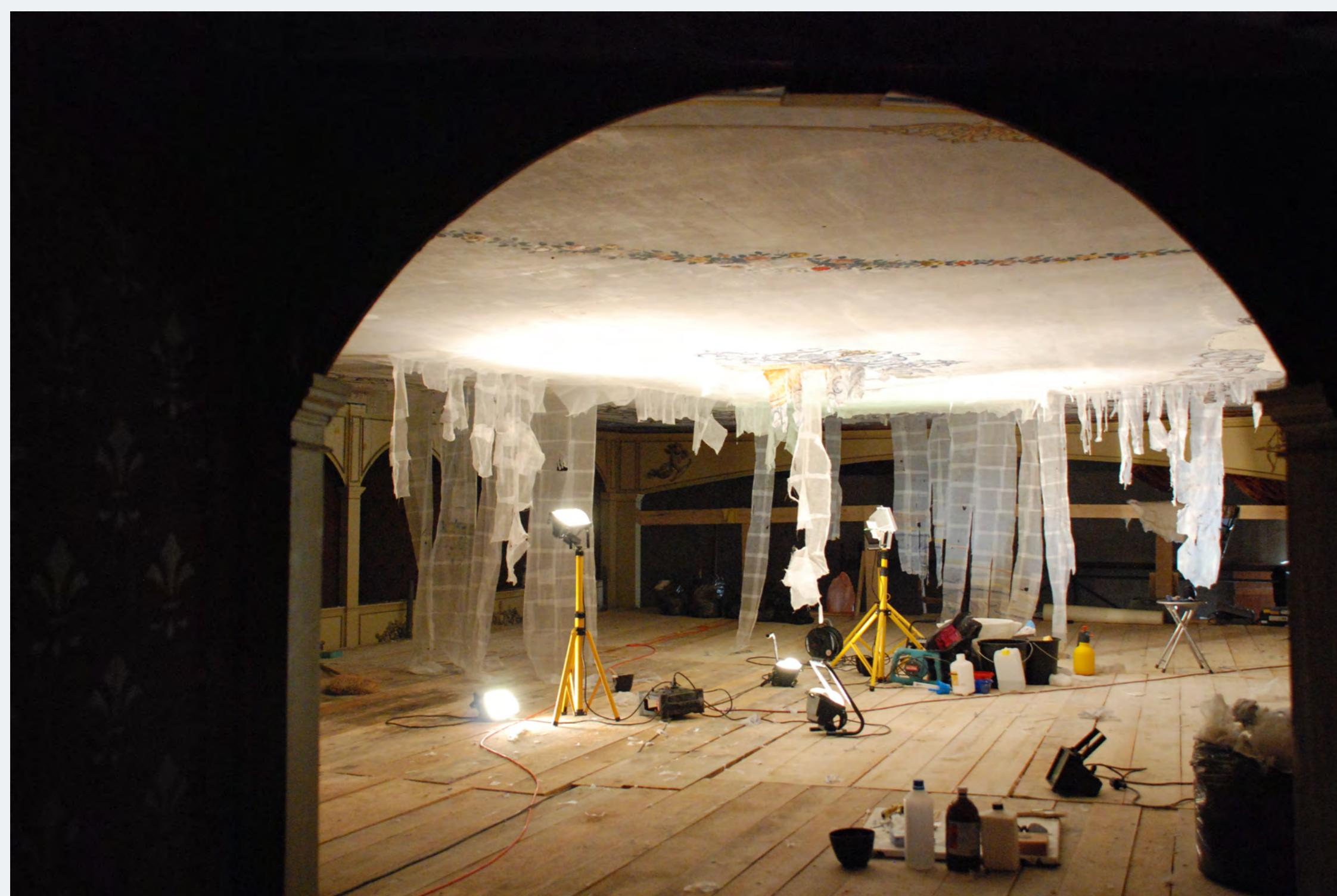
The removal of the facing from a painting consists primarily of dissolving the glue, so that the reinforcing material can easily be removed. The solvent weakens the adhesive capacity of the glue in the facing, and the facing can be removed by gentle pulling.
