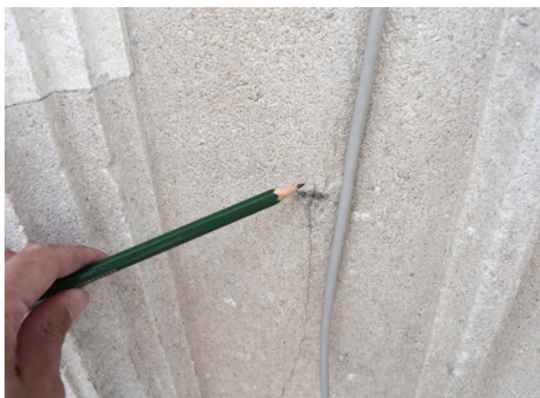
10. Orlando's Column, pillar, east side, vertical crack in 2021 (HRZ Archive, V. Marinković, 2021)
