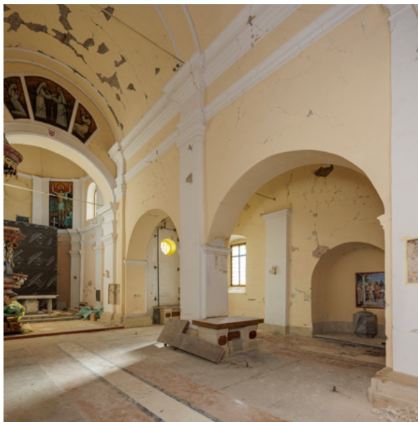
8. Pogled na bočni brod i svetište, stanje tijekom obnove nakon potresa 2020. (snimka: P. Mofardin, 2023.) View of the side aisle and sanctuary, condition during reconstruction after the 2020 earthquake (P. Mofardin, 2023)
