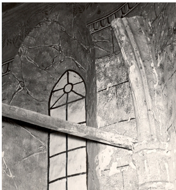
12. Detalj unutrašnjosti – gotički prozori s odbijenim rebrom (Fototeka MKM, 1954., snimka: V. Bradač, inv.br.: 15137, neg.: I-H-103) Detail of the interior: Gothic windows with broken ribs (V. Bradač, MKM Photo Archive, 1954, inv. no.: 15137, neg.: I-H-103)
