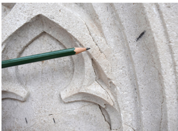
11. Orlando's Column, pillar, east side, unstable damage in 2021 (HRZ Archive, V. Marinković, 2021)
