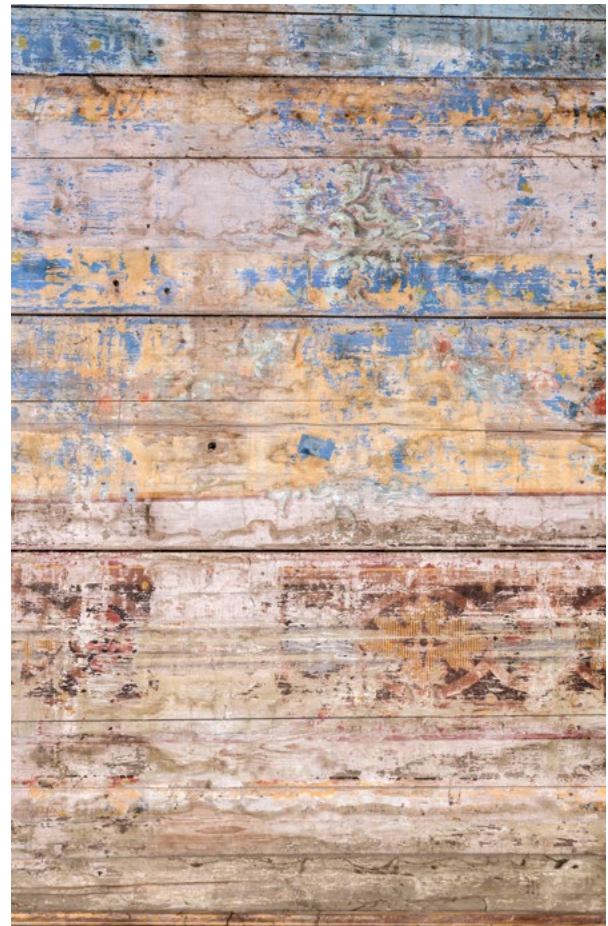
9. Detalj oslikane oplata svoda, kartuše s rokajima i girlandama te tragovima friza s geometrijskim motivima, zatečeno stanje (arhiva HRZ-a, snimka: G. Tomljenović, 2016.) Detail of the painted panelling of the vault, cartouches with rocaille decorations, garlands and traces of friezes with geometric motifs before conservation (HRZ Photo Archive, G. Tomljenović, 2016)
