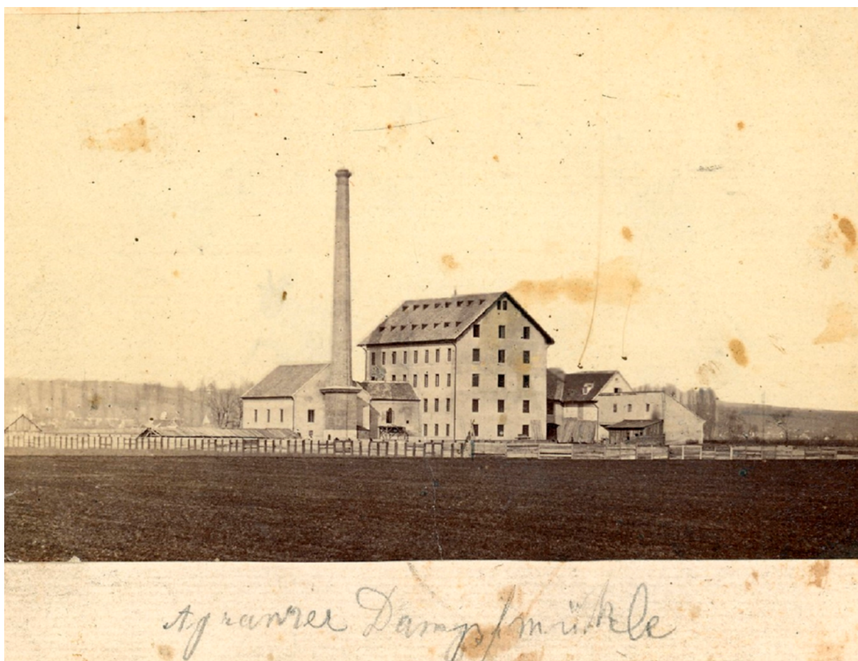
11. Paromlin complex in Zagreb, 1861 (Photo library of Zagreb City Museum, MGZ-fot-6371) Kompleks Paromlin u Zagrebu, 1861. (fototeka MGZ)
