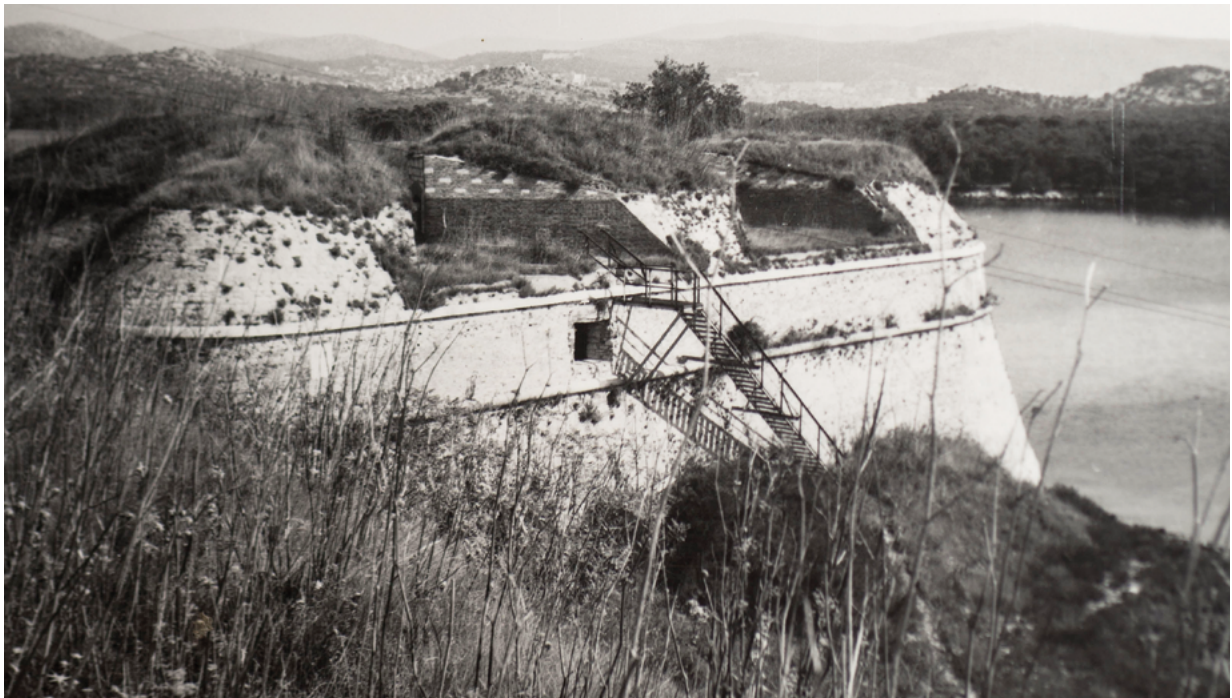
9. Metalno pomoćno stubište uz jugoistočni bastion u rujnu 1971. (MKM-KO ST - F: snimka: S.M., inv. br. 38618, br. neg. L-13786) Metal auxiliary staircase next to the south-eastern bastion, September 1971 (MKM-KO ST - F, S.M., inv. no. 38618, neg. no. L-13786)
