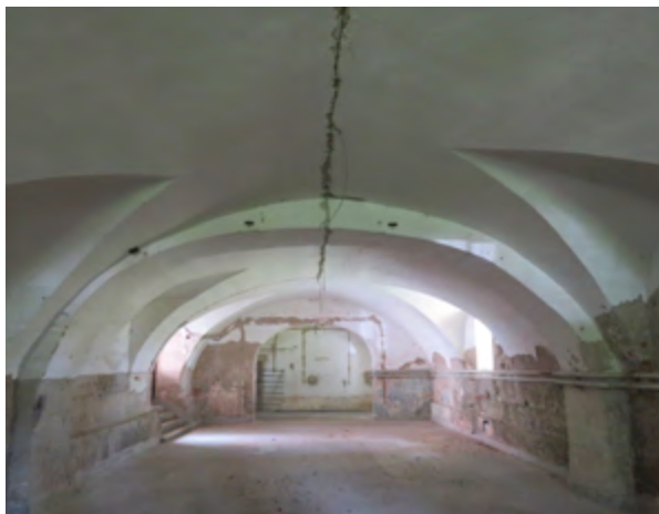
9. Dvorac Kerestinec, bačvasti svod poluukopane prostorije zapadnog krila (snimka: V. Jakaša Borić, 2019.) Kerestinec castle, barrel vault of a half-buried room in the west wing (V. Jakaša Borić, 2019)
