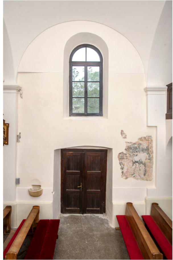
18. Južni zid lađe nakon konzervatorsko-restauratorskih radova (fototeka HRZ-a, snimio J. Kliska, 2018.) South wall of the nave after conservation (Croatian Conservation Institute Photo Archive; J. Kliska, 2018)
