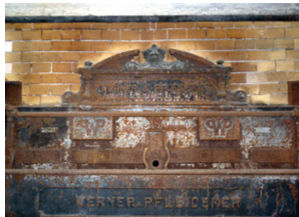
Sl. 14. Detalj sačuvane krušne peći proizvođača Werner & Pflleiderer (fototeka HRZ-a, snimila I. Pauk Sili) Details of the preserved brick oven made by Werner & Pflleiderer (Croatian Conservation Institute Photo Archives, I. Pauk Sili)
