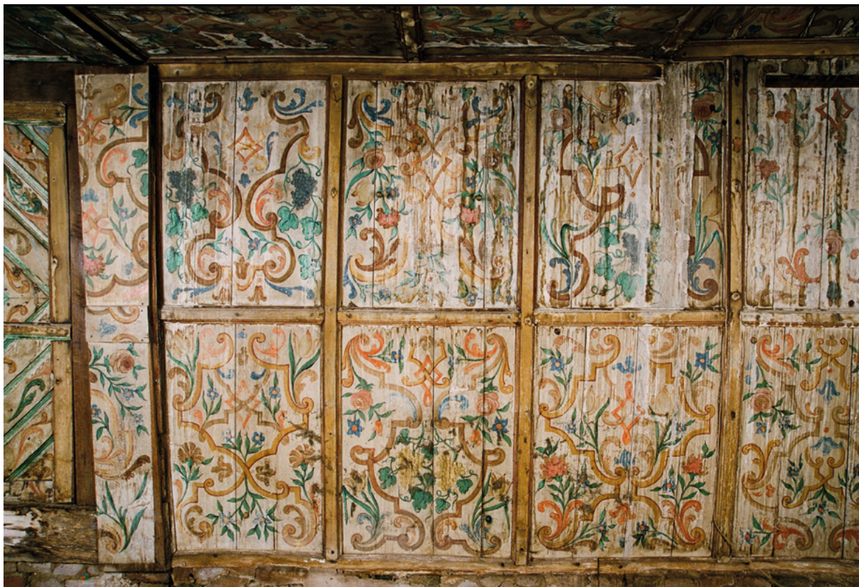
2. Pogled na sjeverni zid lađe prije konzervatorsko-restauratorskih radova (fototeka HRZ-a, snimio V. Barac, 2001.) View of the north wall of the nave before conservation (Croatian Conservation Institute Photo Archive, photo by V. Barac, 2001)
