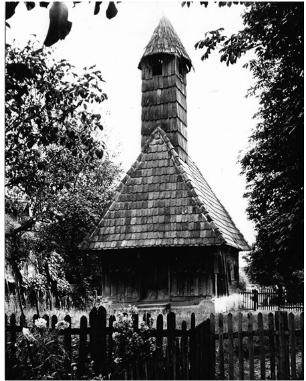
5. Pogled na kapelu nakon zamjene krovnog pokrova biber-crijepom, druga polovica 20. stoljeća (fototeka Instituta za povijest umjetnosti, inv. br. Stb.F-4, snimio I. Nikolić) View of the chapel after replacing the roof covering with beaver tail tiles, second half of 20th c. (Institute of Art History Photographic Collection, inv. no. Stb.F-4, photo by I. Nikolić)
