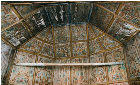
6. Pogled na svod svetišta prije konzervatorsko-restauratorskih radova (fototeka HRZ-a, snimio V. Barac, 2001.) View of the sanctuary vault before conservation (Croatian Conservation Institute Photo Archive, photo by V. Barac, 2001)
