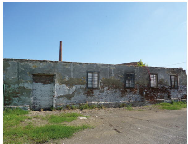
4. Pogled na južno pročelje zatečenog ostatka male Hornwerk vojarne (fototeka HRZ-a, snimila I. Pauk Sili) View of the south front of the Large Hornwerk Barrack remains (Croatian Conservation Institute Photo Archive, photo by I. Pauk Sili)
