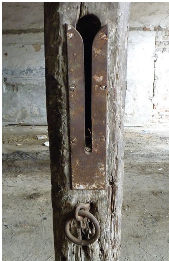
15. Metalni utori na drvenim stupovima konjušnice za ugradnju pregrada (fototeka HRZ-a, snimila I. Pauk Sili) Metal slots for installing partitions on wooden columns in the stables (Croatian Conservation Institute Photo Archive, photo by I. Pauk Sili)
