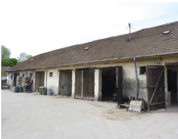
3. Pogled na istočno pročelje velike Hornwerk vojarne (fototeka HRZ-a, snimila I. Pauk Sili) View of the east front of the Large Hornwerk Barrack (Croatian Conservation Institute Photo Archive, photo by I. Pauk Sili)
