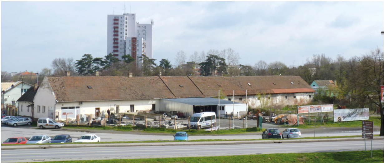
1. Pogled na zapadno pročelje velike Hornwerk vojarne (fototeka HRZ-a, snimila I. Pauk Sili) View of the west front of the Large Hornwerk Barrack (Croatian Conservation Institute Photo Archive, photo by I. Pauk Sili)
