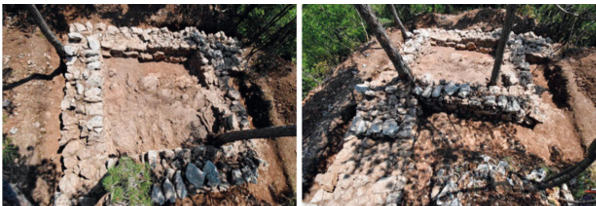
17. Pogled na istražene građevinske strukture na lokalitetu Obrovac - Kalić (snimio T. Percan) View of the investigated buildings at the Obrovac–Kalić site (photo by T. Percan)
