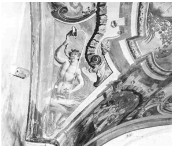
8. Stanje freske na jugozapadnoj peti svoda s vidljivim oštećenjima 1972. godine (Arhiv RZH-a, inv. br. II-15-17, snimio I. Maroević) Condition of the fresco on the southwest foot of the vault with visible injuries in 1972 (former Conservation Institute of Croatia archive, inv. no. II-15-17, photo by I. Maroević)
