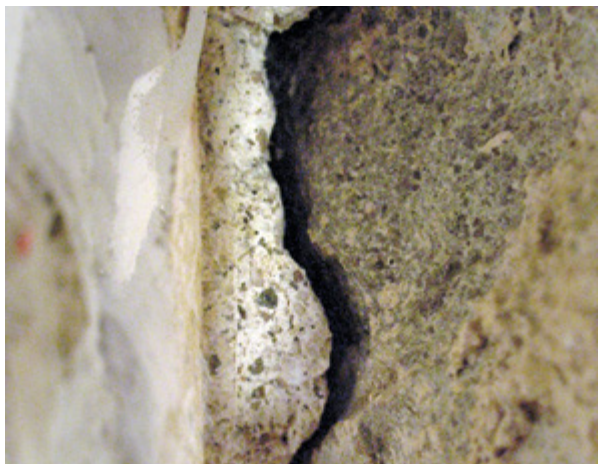
5. Šupljina, odvajanje arriccio od nosača (snimio B. Hacker, 2009.) A cavity, arriccio detaching from the support (photo by B. Hacker, 2009)
