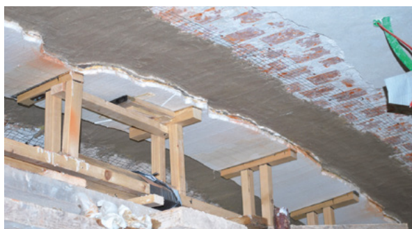
15. Detalj fragmenta nakon žbukanja armature mrežice (snimio M. Jelenčić, 2010.) Detail of the fragment after plastering the armature grid (photo by M. Jelenčić, 2010)
