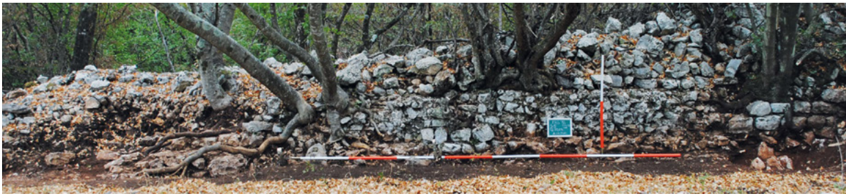
6. Remains of the eastern wall of the Late Antique complex (SU 059) (Croatian Conservation Institute Photo Archive, photo by A. Janeš, 2012) Ostaci istočnog zida kasnoantičkog kompleksa (SJ 059) (fototeka HRZ-a, snimio A. Janeš, 2012.)
