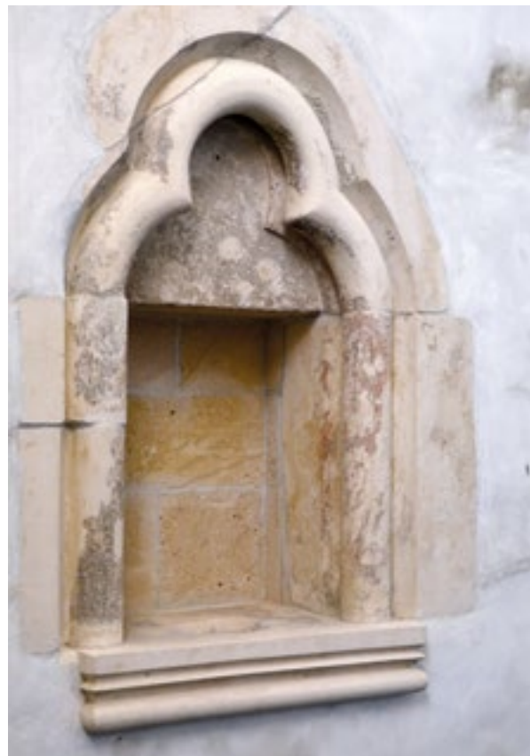
14. Gora, crkva Uznesenja BDM, sakrarij u južnom zidu svetišta nakon ponovne ugradnje (snimio D. Miletić). Gora, Church of the Assumption of the B. V. Mary, sacrarium in the southern wall of the sanctuary, after it was re-embedded (photo by D. Miletić)
