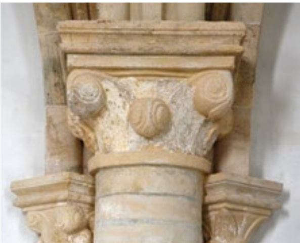
24. Gora, crkva Uznesenja BDM, kapiteli polustupa J3 (snimio D. Miletić). Gora, Church of the Assumption of the B. V. Mary, capitals of the half-column J3 (photo by D. Miletić)
