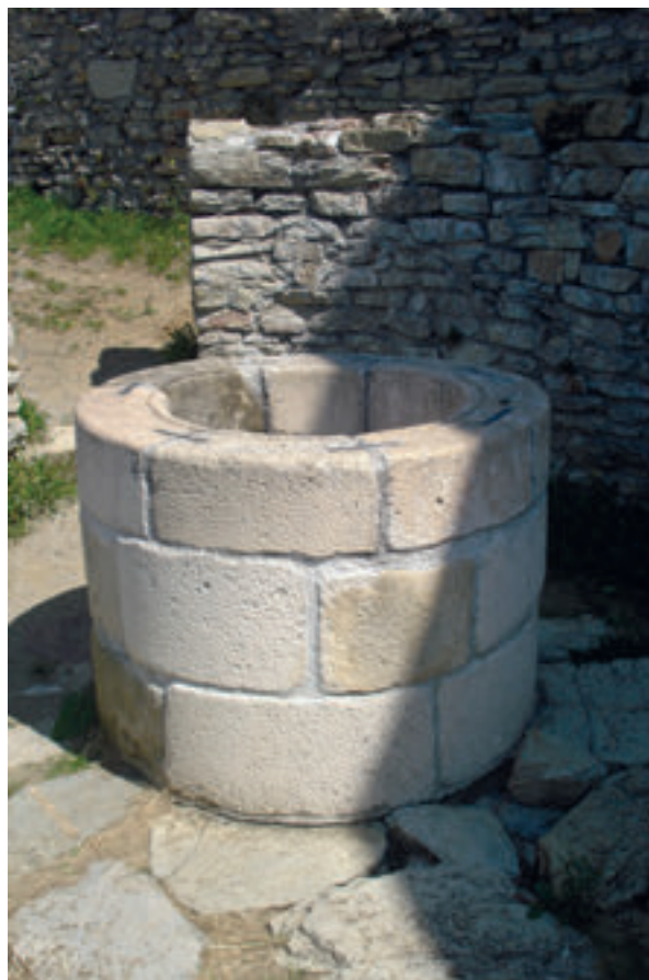
14. Kruna vodospreme rekonstruirana je s tri reda isklesanog prirodnog i umjetnog kamena, a elementi najgornjeg reda spojeni su brončanim skobama (snimio H. Malinar). The crown of the reservoir was reconstructed in three tiers cut from natural and artificial stone, with elements of the top tier held together by bronze clamps (photo by H. Malinar)
