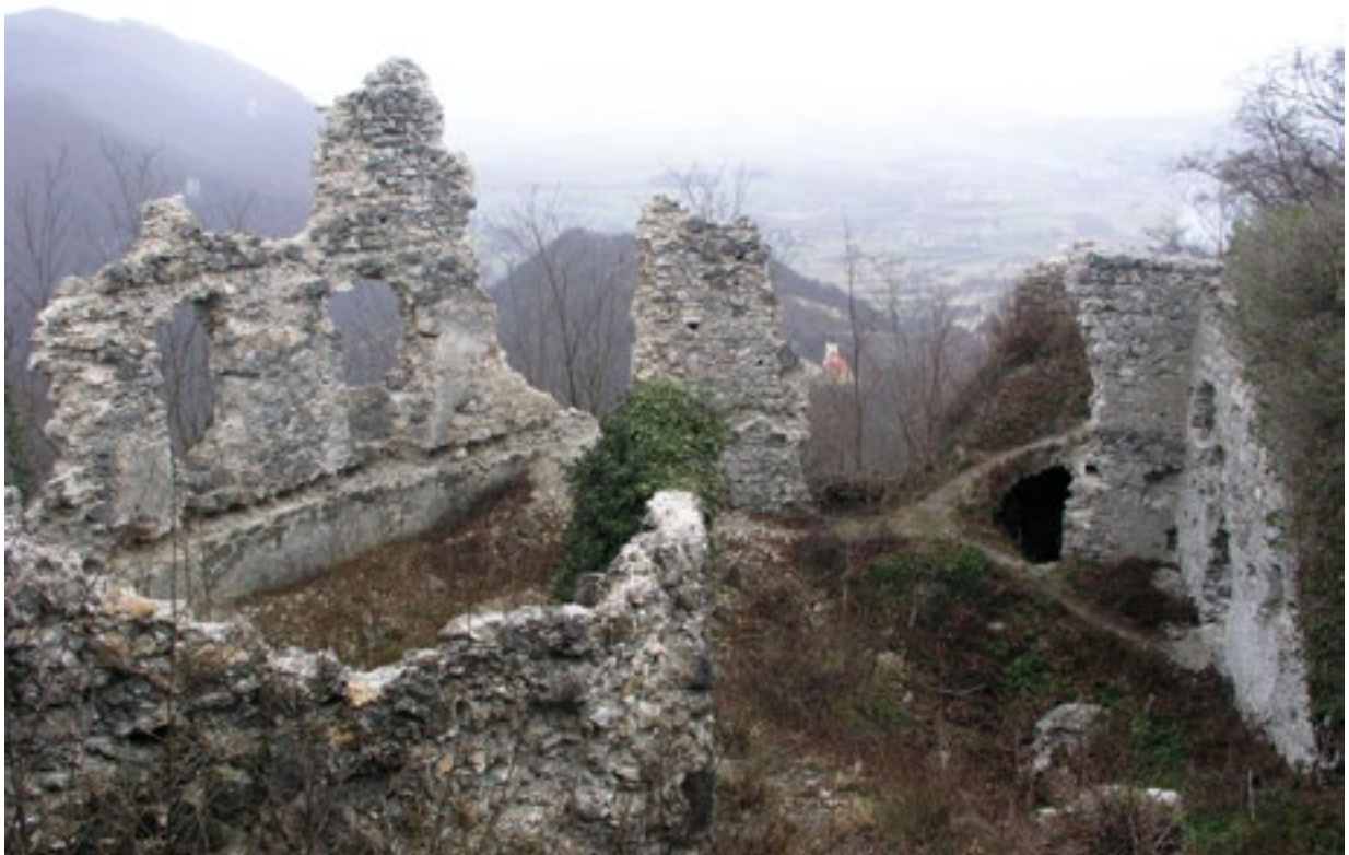
5. Pogled na središnje dvorište i južno krilo palasa K (fototeka HRZ-a, snimio R. Čimin, 2008.). View of the central courtyard and the southern wing of the Great Hall K (Croatian Conservation Institute Photo Archive, photo by R. Čimin)
