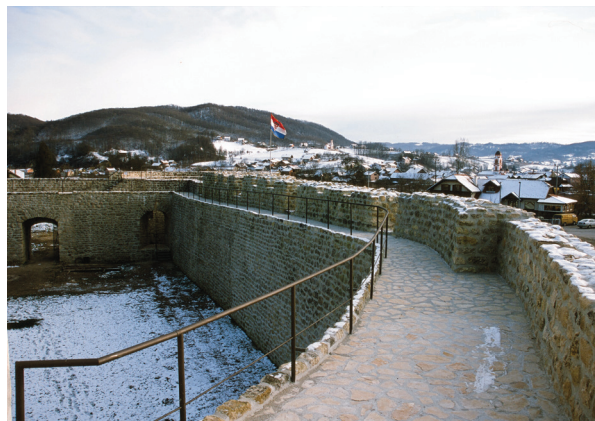
21. Krunište južnog obrambenog zida nakon radova The parapet of the southern defense wall after restoration
