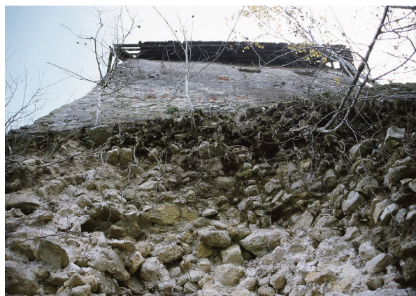
18. Kostajnica, Stari grad, urušenje obrambenog zida ispod peterokutne kule Kostajnica, Old Town, the collapse of the defensive wall below the pentagonal tower
