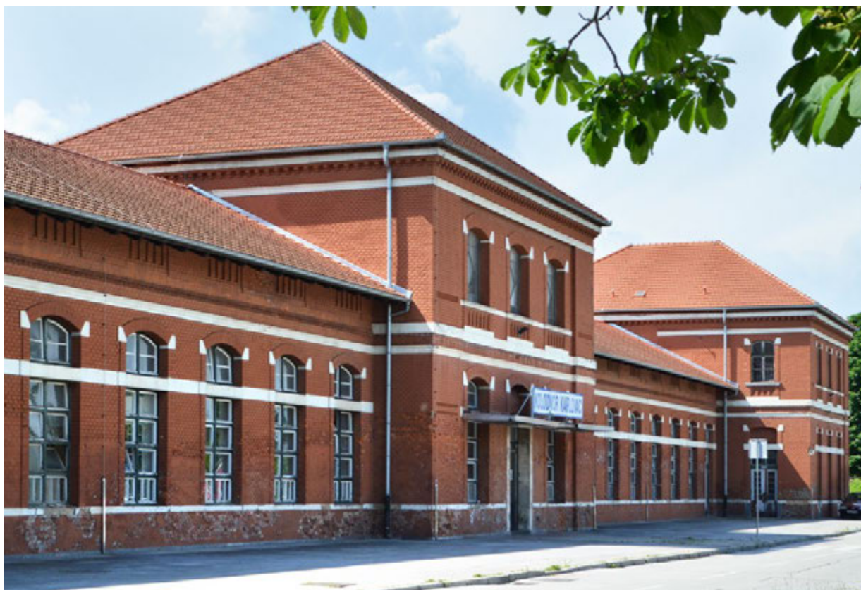
8. Prijemna zgrada kolodvora Hrvatskih željeznica u Karlovcu 2019. (snimka D. Damjanović, 2019.) Reception building of the Croatian Railways station in Karlovac in 2019 (D. Damjanović, 25 May 2019)
