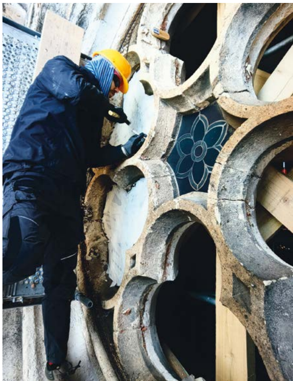
17. Stanje tijekom demontaže vitraja glavne apside (Bokart d.o.o.) Condition during dismantling of the stained-glass window in the main apse (Bokart)
