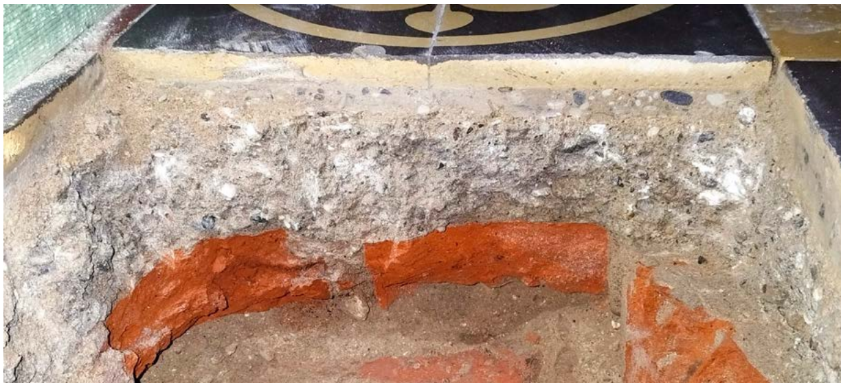
18. Stratigrafija podne obloge s keramitnim pločicama u brodovima katedrale (arhiva HRZ-a, snimka: T. Šaina, 2022.) Stratigraphy of the floor covering with ceramic tiles in the naves of the cathedral (HRZ Archive, T. Šaina, 2022)
