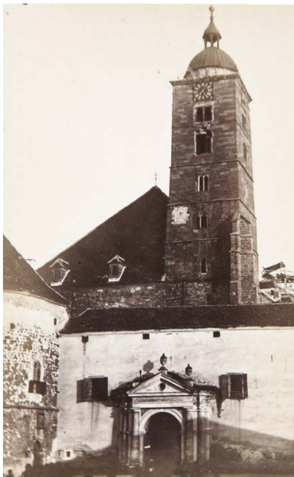
8. Zagrebačka katedrala unutar renesansne tvrđave, pogled na klasicistički portal uz Bakačevu kulu, nakon potresa 1880. (MGZ, inv. br. fot-15857/11, snimka: H. Fickert, 9. studenoga 1880.) Zagreb cathedral inside the Renaissance fortress, view of the classicist portal next to the Bakač Tower, after the earthquake of 1880 (MGZ, inv. no. fot-15857/11, H. Fickert, 9 November 1880)
