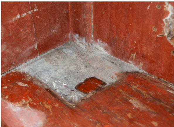
16. Unutrašnjost donjeg dijela ormara, tijekom kemijsko-mehaničkog čišćenja (fototeka HRZ-a, snimio D. Gazde, 2010.) Interior of the lower part of the cabinet, during chemical and mechanical cleaning. (Croatian Conservation Institute Photo Archive; D. Gazde, 2010)
