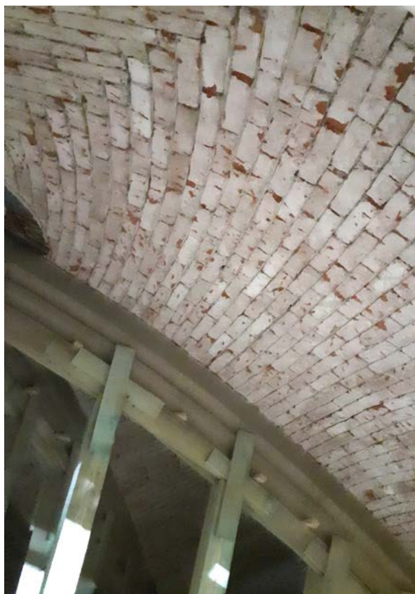
21. Pogled na svod izgrađen nakon potresa 1880. (fototeka GZZSKP-a, 2023.) View of the vault built after the 1880 earthquake (GZZSKP Photo Archive, 2023)
