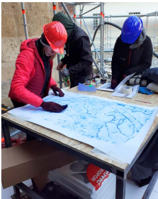
17. Označavanje i dokumentiranje vrste i razine oštećenja vitraja nakon demontaže proveli su djelatnici tvrtke Bokart d.o.o. (fototeka GZZSKP-a, 2023.) Marking and documentation of the type and level of damage to the stained glass after dismantling was carried out by employees of the company Bokart (GZZSKP Photo Archive, 2023)
