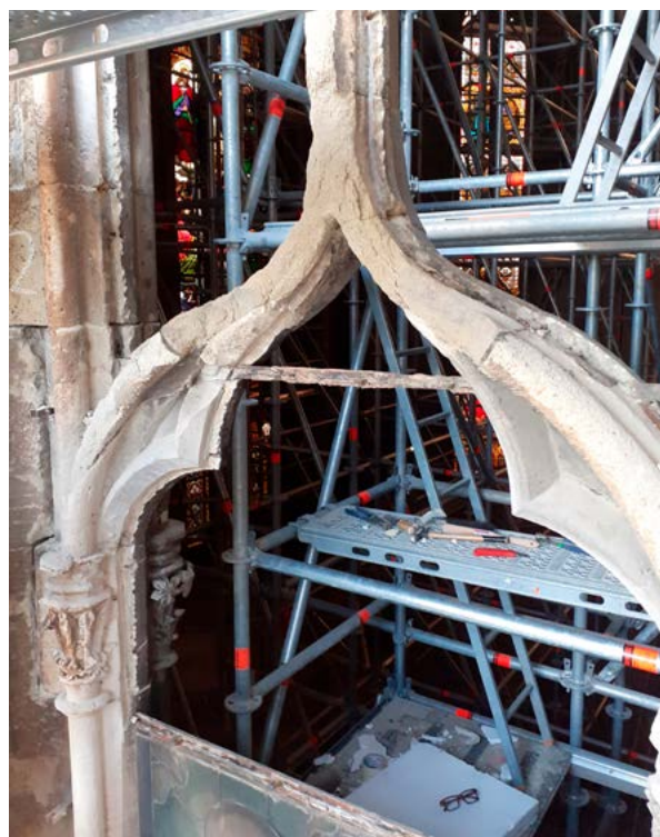
18. Dotrajali kameni prozorski profili i tzv. sedlo od kamena pješčenjaka (fototeka GZZSKP-a, 2023.) Dilapidated stone window profiles and the so-called saddle of sandstone (GZZSKP Photo Archive, 2023)
