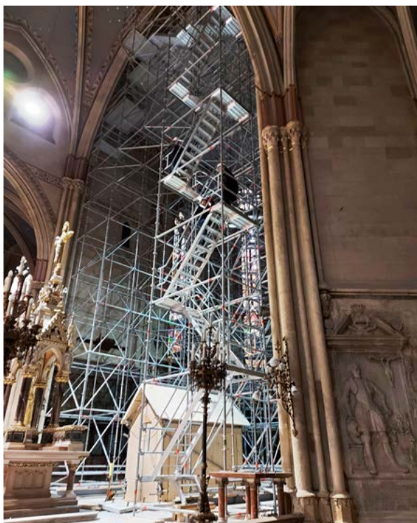
10. Pogled iz južnog broda na izrađenu drvenu oplatu za grob bl. Alojzija Stepinca (fototeka GZZSKP-a, 2021.) View from the south aisle of the wooden coverings for the tomb of the Blessed Aloysius Stepinac (GZZSKP Photo Archive, 2021)
