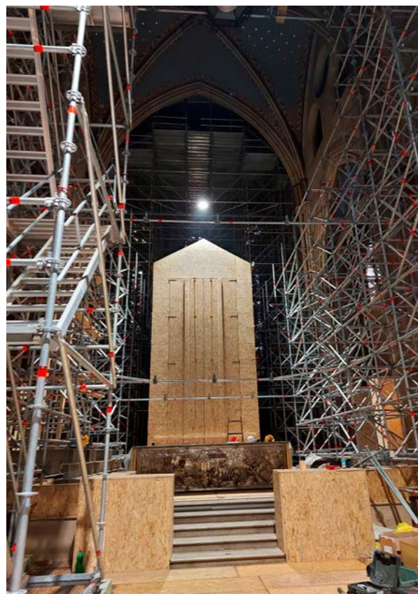
13. Glavni oltar katedrale tijekom zatvaranja u drvenu oplatu (fototeka GZZSKP-a, 2022.) Main altar of the cathedral during its enclosure in wooden coverings (GZZSKP Photo Archive, 2022)
