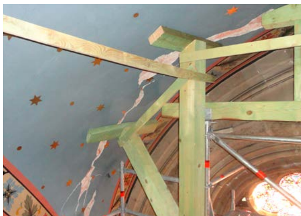
9. Drvene podupore svoda svetišta (fototeka GZZSKP-a, 2021.) Wooden supports of the sanctuary vault (GZZSKP Photo Archive, 2021)
